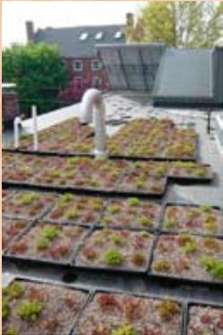
The roof garden helps insulate the building, and, with planted seedum, reduces storm water runoff.
